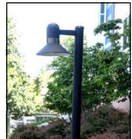
Full cut-off lighting fixture.
