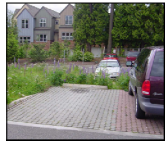
Parking area constructed of grid pavers.
